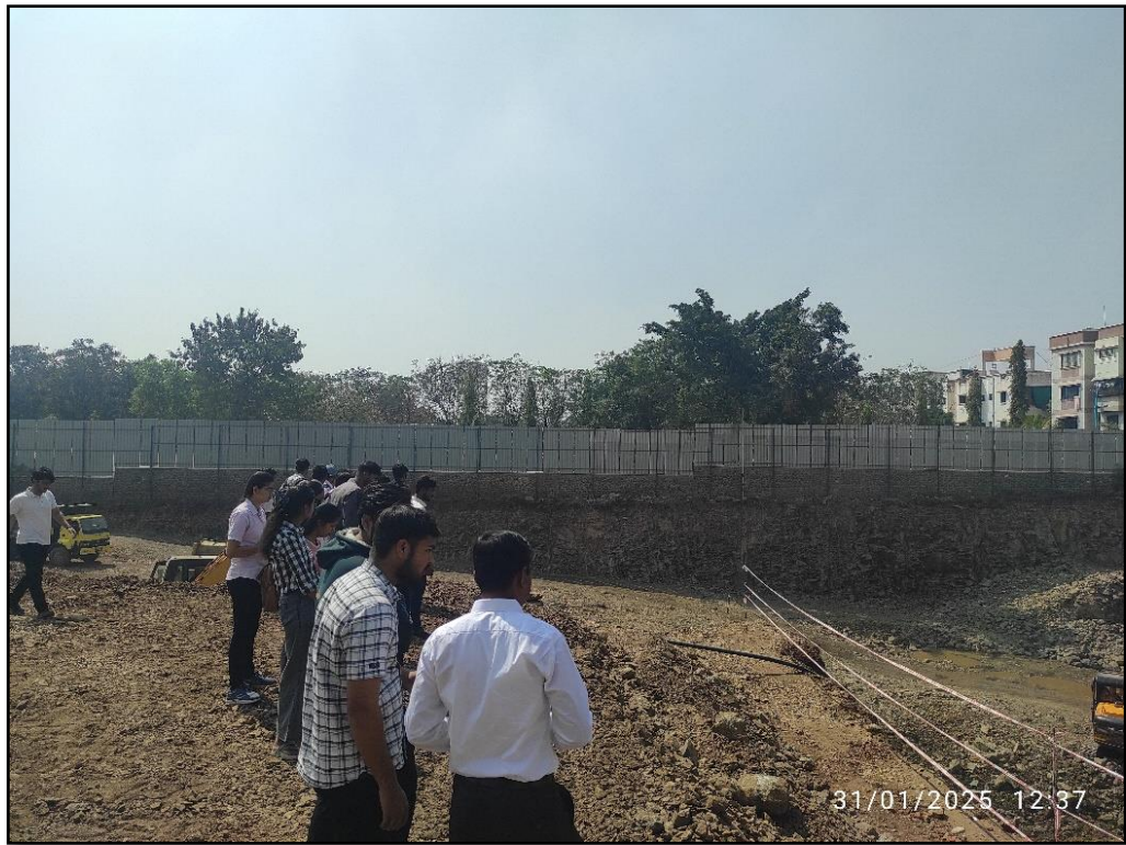
Fig. 5: students watching ongoing construction activities and understanding site layout, plan for execution of project.
