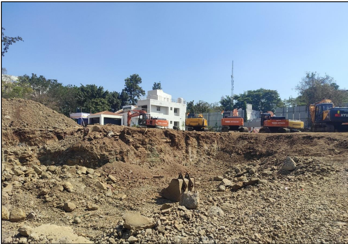
Fig.7,8: Excavation on site for foundation and construction of Building A
